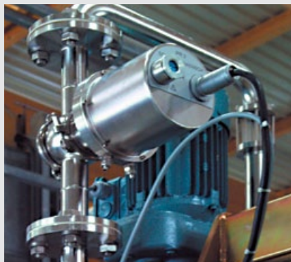
Inline installation (with bypass for maintenance work) Installation in circulating process with pump
